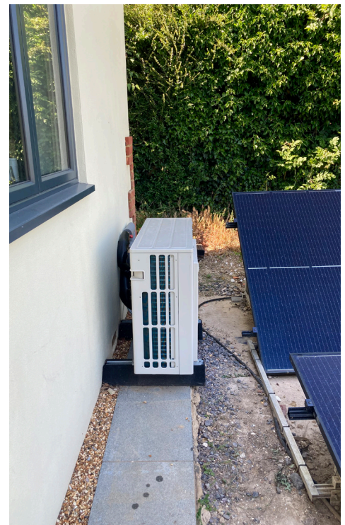
Fig. 3 Air source heat pump linked to underfloor heating system
