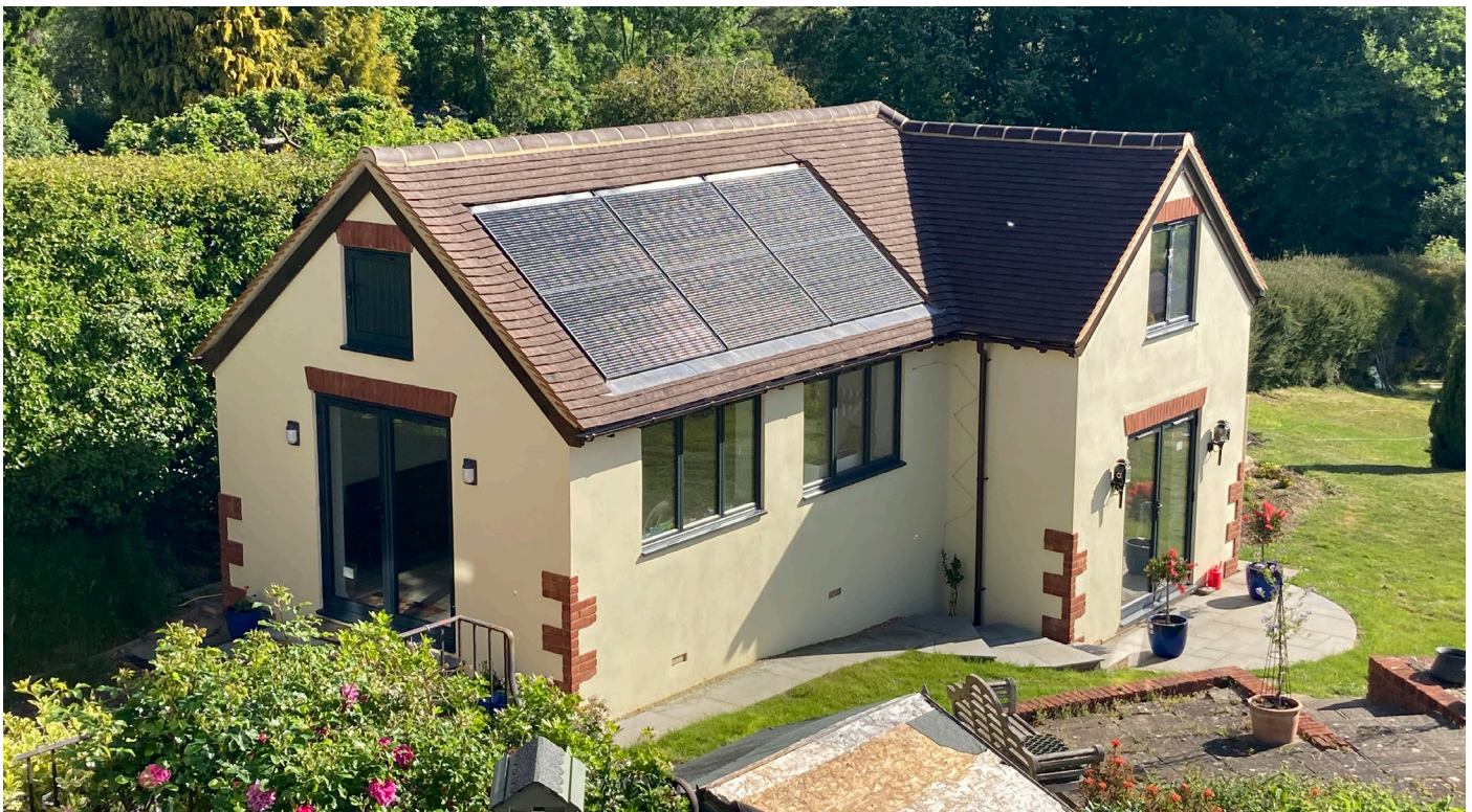
Fig. 1 Eco house with triple glazed doors and windows. Photovoltaic solar panels built into roof.
